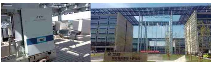
Guodian 2.58MW Photovoltaic Project in Beijing
