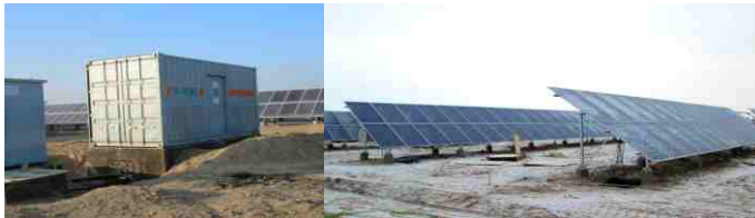
30MW PV Project in Xinjiang Production and Construction Corps
