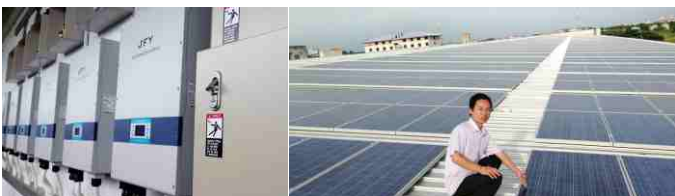
1.2MW Rooftop Distributed PV Project in Bangkok, Thailand
