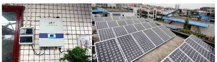
The First 10kW Household PV Project in Sichuan
