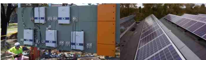
100kW PV Project in Sydney, Australia
