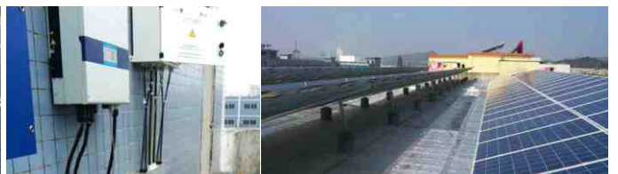
12kW Distributed Photovoltaic Project in Huaihua
