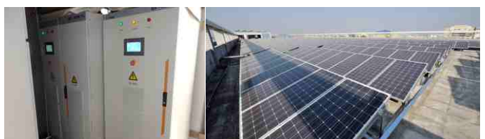
1.5MW Distributed Generation Project in Hohhot Middle School
