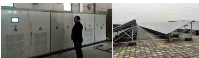
1MW Rooftop PV Project in Jiangsu Electric Power
