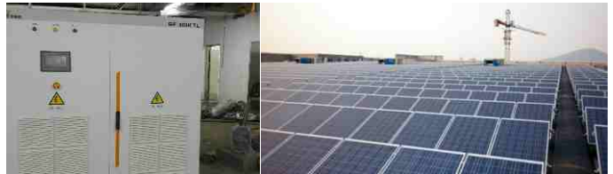
6.5MW Photovoltaic Grid Project in Hefei
