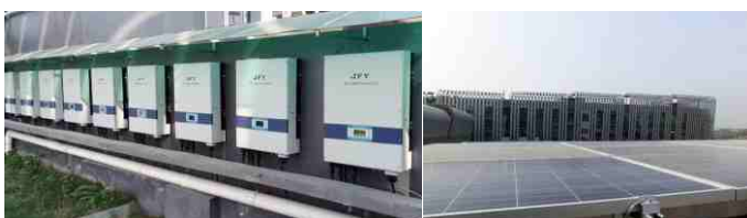
500kW On-grid PV Project in Shenzhen North Railway Station
