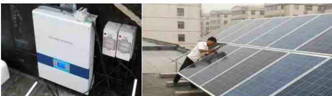
10kW Distributed Photovoltaic Project in Handan
