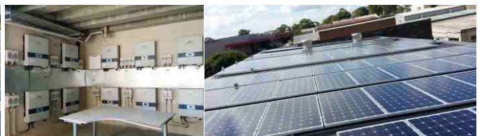
100kW PV Project in NSW, Australia
